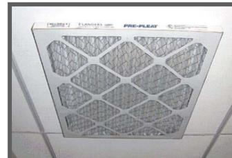
**Pathway Interruption:** MERV 8 Filter installed during construction
