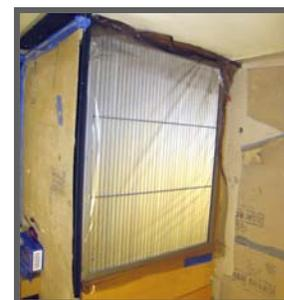
**HVAC Protection:** Duct equipment sealed with plastic
