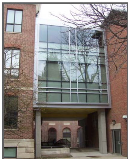
New Connector between Mallinckrodt and Conant Photo: JBM General Contractors, 2009
