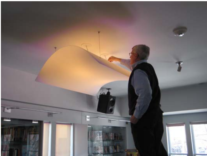
OFS and FMO commissioning the space Photo: OFS
