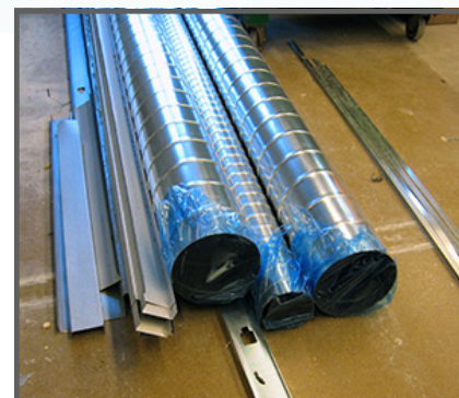
IAQ Management HVAC Protection: Ductwork kept sealed before installation
