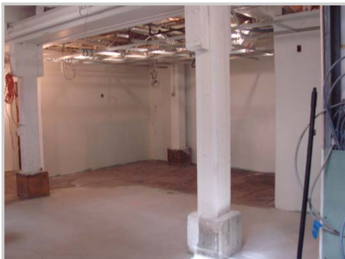
Construction in progress Photo: Harvard Green Building Services, 2010
