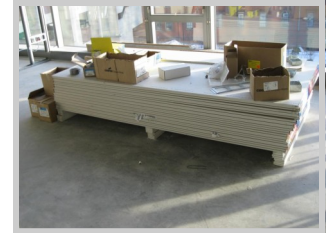
Porous materials were stored raised up off the floor on dunnage.
