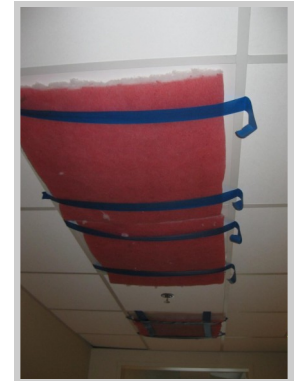
Supply and return diffusers were covered with MERV 8 filtration media.
