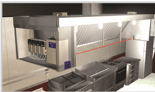
Melink VAV Kitchen Hood Exhaust: copyright Melink, 2013
