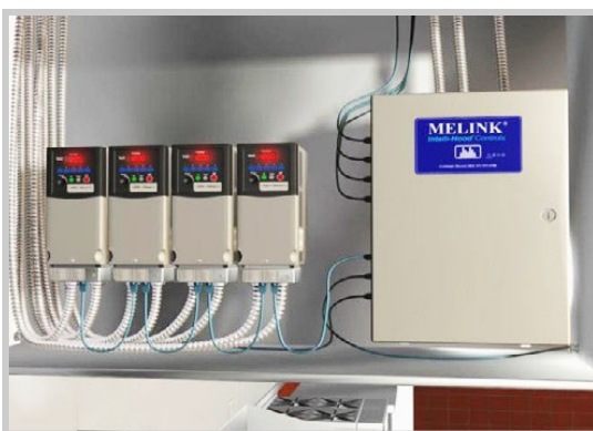
Melink Kitchen Hood Exhaust Controls: copyright Melink, 2013
