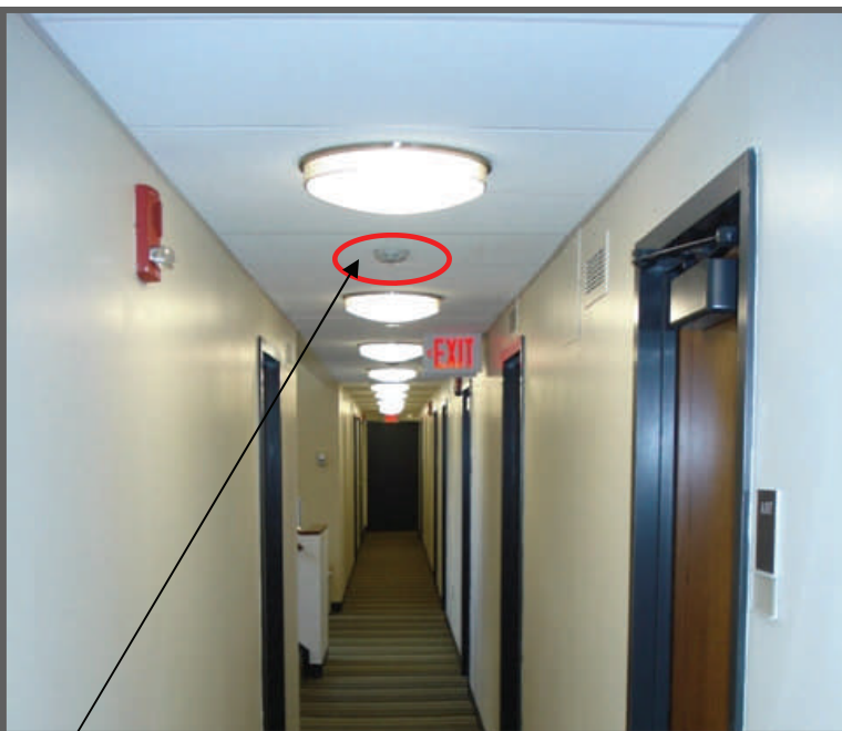
Occupancy Sensors in McCulloch Hall corridors
