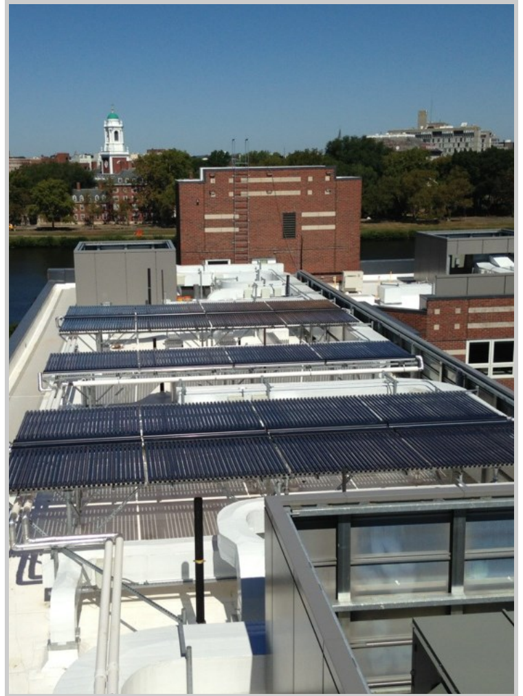
Rooftop Solar Thermal System—Photo Copyright Kingspan Environmental 2015
