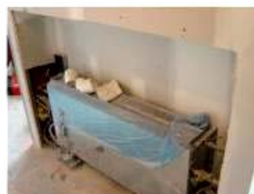
2/28/08 Covered Unit Heaters
