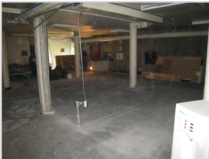
A Clean Construction Site
