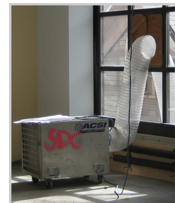
Pathway Interruption: Exhaust filtered and direct to outside
