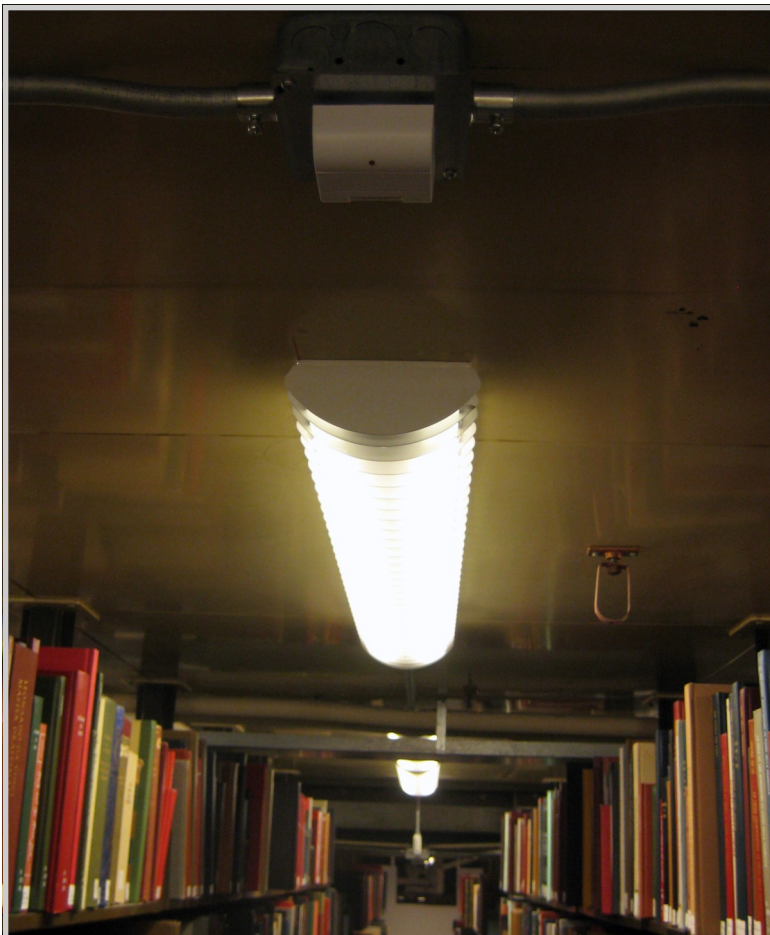
<-Occupancy Sensors (Top) in Stacks Photo: Harvard Green Building Services
