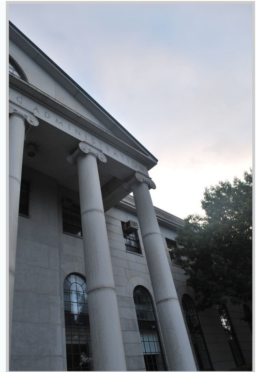
Littauer Front Entrance Photo: Harvard Green Building Services
